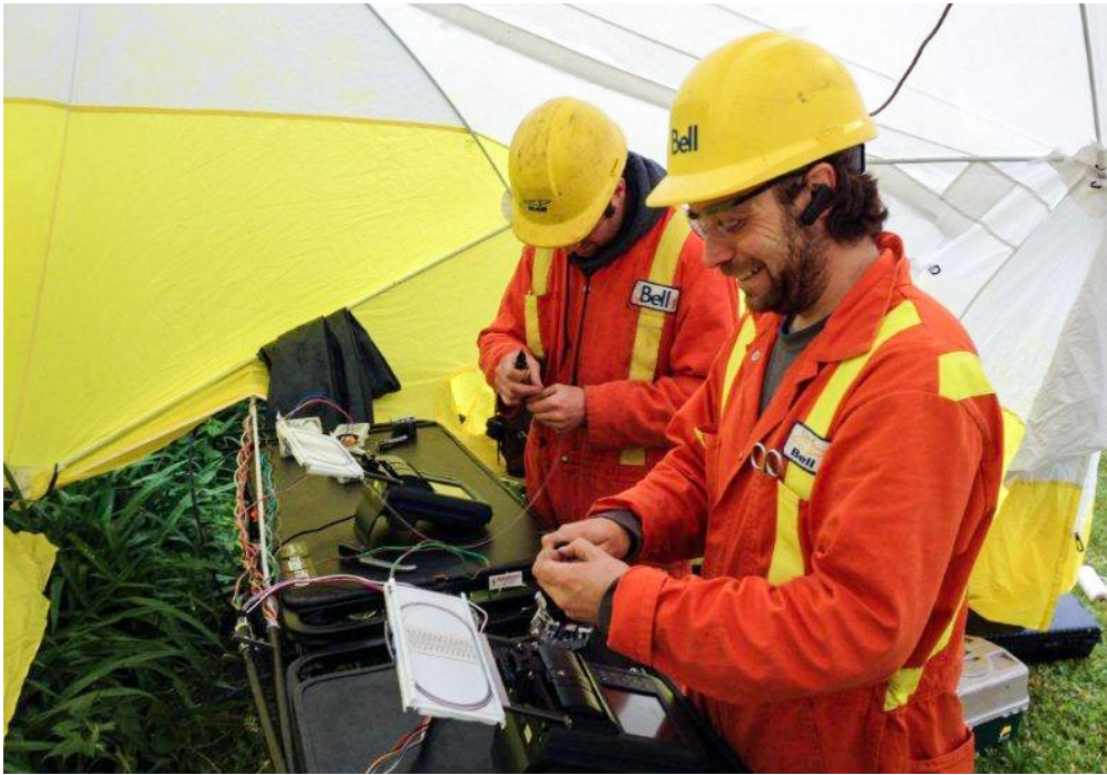
Bell team members experimenting with a squirrel repellent to protect the sheaths of fibre optic cables.
