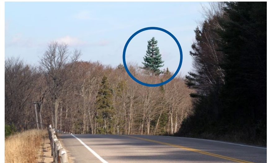
Bell certifies that all its antenna base-station installations or towers meet or exceed federal Safety Code 6 requirements. In this picture a tower is disguised as a tree and is positioned to blend with the environment.
