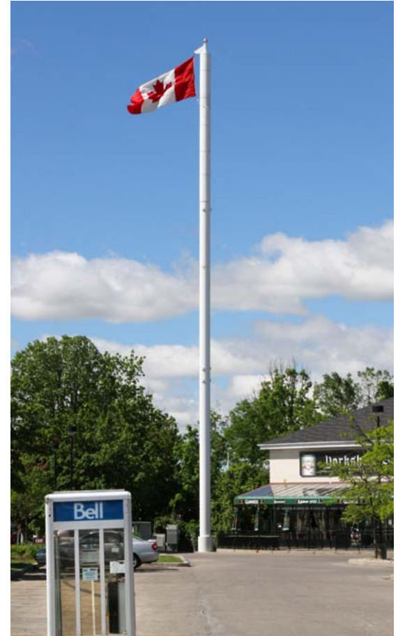
A Bell Mobility antenna built within a flagpole
