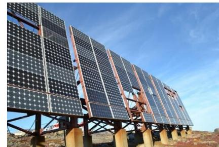
To maintain the service in remote areas, cell sites rely on diesel-powered generators, which run fulltime and emit important amounts of GHG emissions and other pollutants. By installing photovoltaic panels to generate electricity and stocking surplus in batteries, generator runtime—and thus fuel consumption—is reduced significantly.
