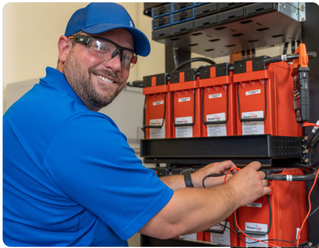
Bell team member proactively setting up back up power generators
